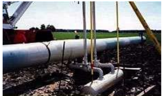
A 26" piggable drip is installed in 1996 on the Union Gas Ltd. natural gas storage and transmission system at the Dawn compressor station near Chatham, Ontario. Union's system handles more than 1.2 tcf/year of gas, linking natural gas from Western Canadian and U.S. supply basins to central Canadian and Northeast U.S. markets.
