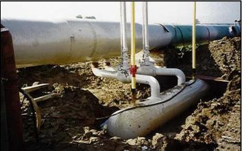
separation technology in a vessel 5X the diameter of the pipeline, expensive and not piggable.
